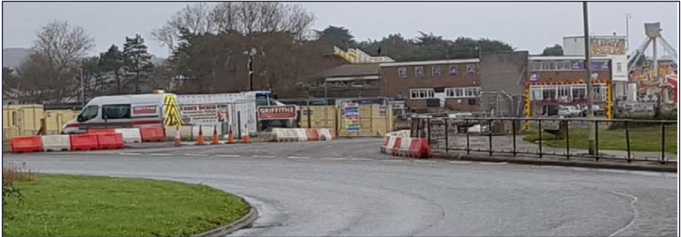
Photo 21 – Existing Access of the A4016 Roundabout
